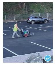
McNears Beach Park parking lot repaying replaced 50-year-old aging asphalt, widened vehicle entries, and improved stormwater runoff.
