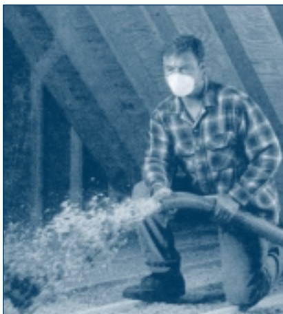
Spray Cellulose Insulation
