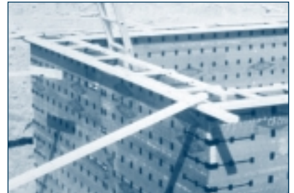
Insulated Concrete Forms (ICFs)
