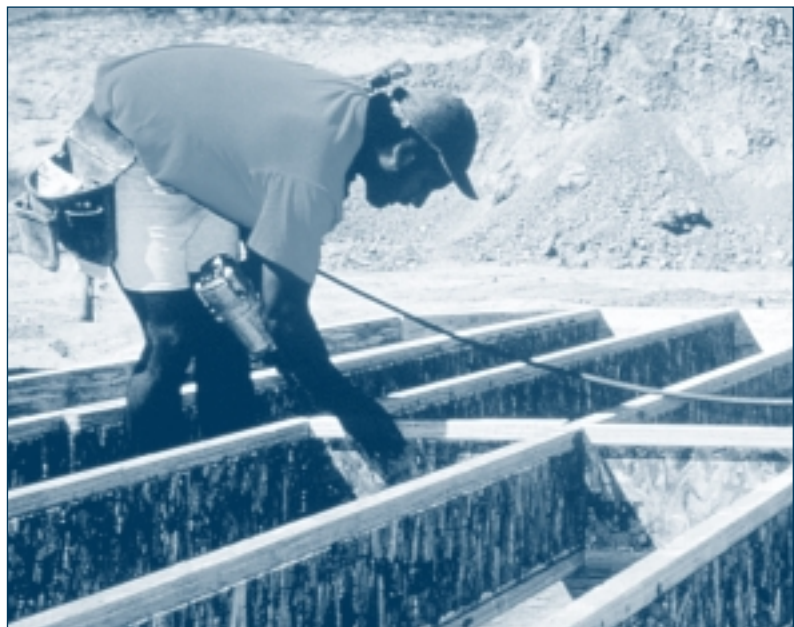
Engineered Wood I-joist
